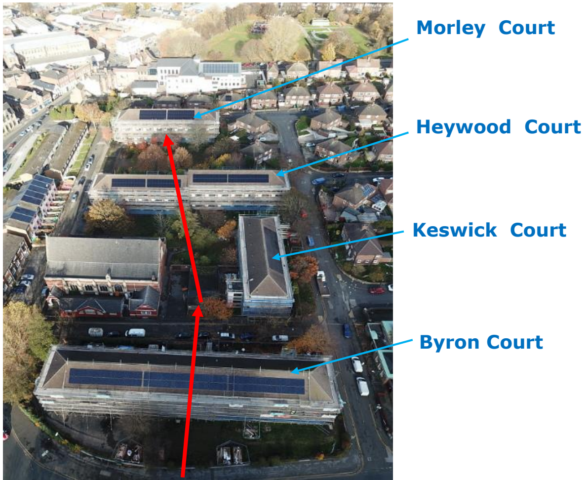
Figure 5: Layout of the Courts and Path of the District Heating Link
