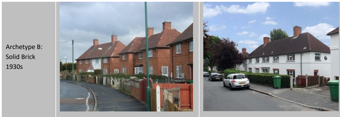
Figure 4: Solid Wall Insulation Example – Before and After
