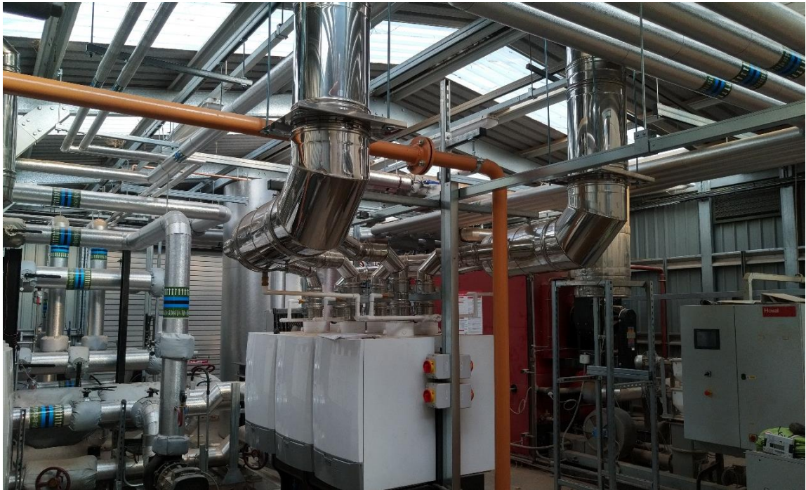
Inside the Combined Heating Plant at Brackenhurst Campus
