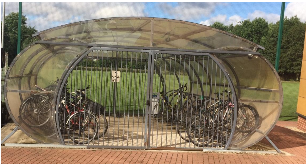
Figure 7 - Typical cycle compound on Clifton
