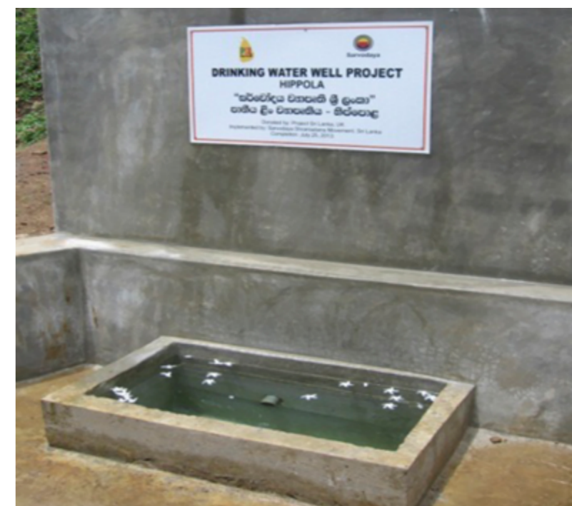
Figure 5: After the Project New Water Well, Hippola Village, Sri Lanka.
