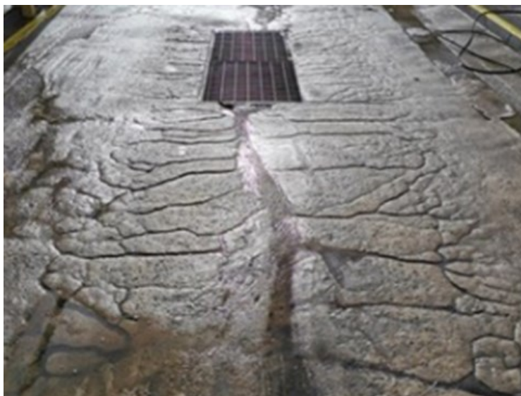
Figure 1. Purpose made water drainage by the petrol station. Surface has been degraded by chemicals
