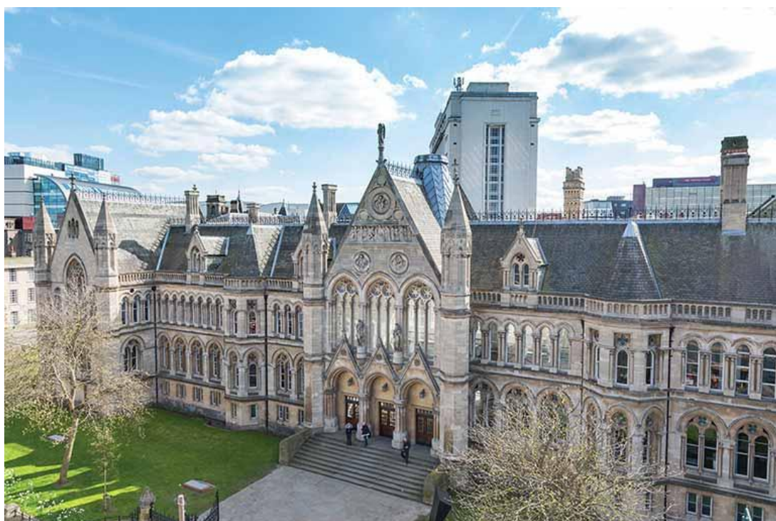
Figure 3 – Arkwright & Newton Buildings
