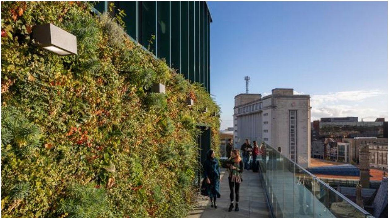
Figure 6 – Design and Digital Arts Building Green Wall
