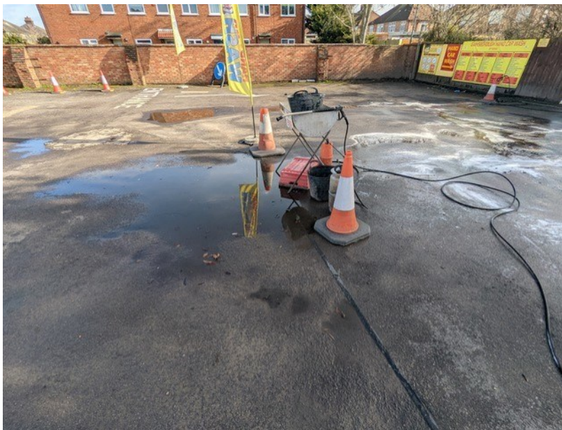
Figure 11: Pooling at a hand car wash, the surface is not designed to handle capacity. Suffolk
