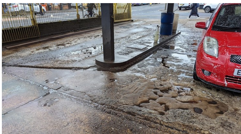
Figure 15: Wash pad with severe corrosion due to use of cleaning chemicals including acid. Leicester
